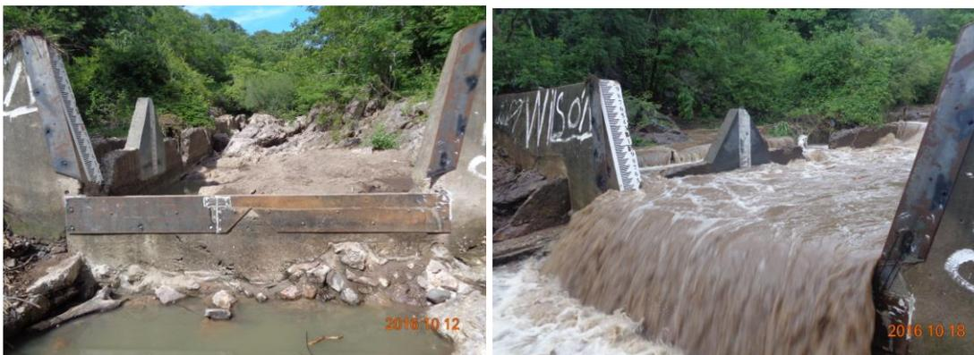
**Figure 3-2: La Simona v-notch weir repair on 12 October 2016 and subsequent flood event on the 18 October 2016**
