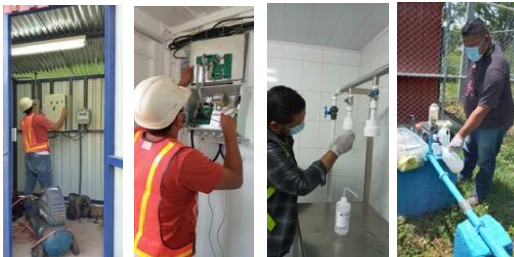
Figure 11: First preventive maintenance of the water treatment plant
