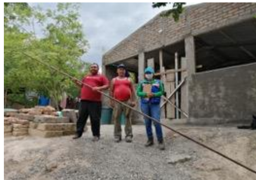
Figure 1: Delivery of materials for the repair of El Bordo temple.
