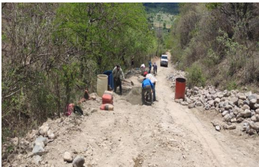
Figure 40: Manual repair of critical points on the road to the communities of El Tanque, Talpetate and El Capulín
