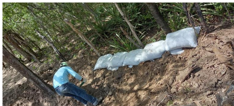
Remediation of platforms and delivery of plants to land owners.
